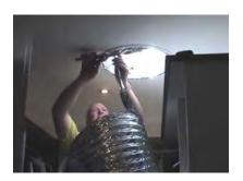
Reach through the Ceiling Frame and pull the Flexitube through the Ceiling Frame and into the room. Continue pulling until it is tight, the wires will lock onto the lip at the top of the Ceiling Frame. Cut the Flexi-Tube off level with the bottom of the Ceiling Frame.
