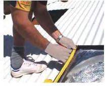
If Sky Tunnel is not being Installed under the Ridge Capping. Measure and Mark approx 90mm down from the back edge of the Soaker Tray, on both sides. Measure and Mark 60mm in from both the side edges along the back edge.
