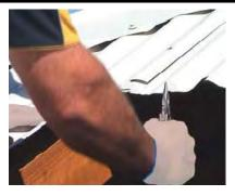
Bend both sides of the cut downwards, to create an overlap, which closes off the corrugations on the high side.
