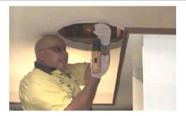
Insert the ceiling frame and attach with the 50mm supachip screws and plastic lugs provided. The plastic lugs are placed on the top side of the ceiling. Fasten the screws through the holes in the ceiling frame, the ceiling and into the white plastic lugs tighten. SEE STEP 5 BEFORE PUTTING IN SCREW CAPS
