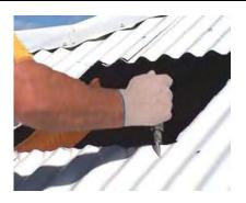
On the low side of the hole, bend up all of the lowest points on the corrugations to prevent any water blowing back up the corrugations, and under the Soaker Tray into the roof space.
