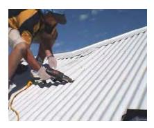
Cut out along the lines that were marked, ensuring cuts finish on the highest point of a corrugation. Ensure the correct cutting tools are used for the roof sheeting., whether manual or electric.
