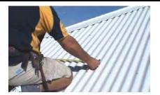
For each Sky Tunnel, double check all your measurements on the roof and the soaker tray to ensure you will get full coverage over the hole, with plenty of overlap on all sides. back of soaker Tray will be under the roof sheets.
