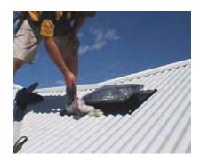
Using a hammer, and rag to protect the surface gently tap the front of the soaker tray between the high points on the roof sheeting to mould the soaker tray to the roof profile.
