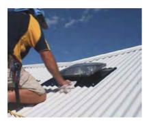
Clean around the Sky Tunnel and the Flashing, removing any Debris and Rubbish from the roof. Be sure to make sure any "swarf" from drilling the metal surfaces is removed to prevent them rusting on the surface of the Soaker Tray or Roof Sheeting.
