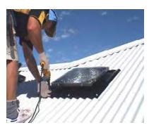
Re-install any Roof Sheeting Tek Screws that were removed. If necessary, these can be fixed through the Soaker Tray.
