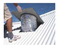
Lower the Sky Tunnel into position. Be careful to make sure the Flexi-tube does not catch on the Roof Sheeting. The back edge of the Soaker Tray will be fitted under the Roof Sheeting. The Soaker Tray should be pushed up until the corners of the Soaker Tray meet flush with the cut in the Roof Sheet.
