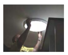
Fit the diffuser into position. Ensure you line up the magnets in the diffuser holder with the magnets on the face of the ceiling frame. If the Sky Tunnel is vented, place the extra magnets provided as a spacer between the diffuser holder magnets and ceiling frame magnets.
