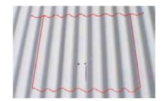
After finding your screw which acts as a guide for the centre of your hole. Mark the Hole Size, it should be approx: 457mm dia - 690mm(w) x 580mm (h) The line along high side should go one corrugation further on both sides, and stop at the highest point of the corrugation. Side lines should also be on highest point.
