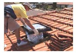
Lower the Sky Tunnel into position. Be careful to make sure the Flexi-Tube does not catch on any of the tiles or roof timbers.
