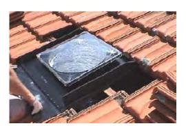
Ensure the rear portion of the soaker tray is underneath the tiles behind and the front portion is on top of the tiles. Re install any tiles (trim if necessary) to cover the sides of the soaker tray.
