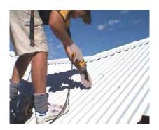
Remove any Roof Sheeting tek Screws from the area around where the Sky Tunnel is going to be installed.
