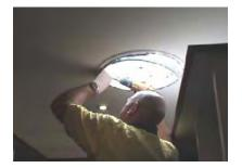
Fit the White Plastic Flexi-Tube locking ring into position with the countersunk screws provided. Start at one end, and work your way around the locking ring. Be sure to line up the 2 x recesses in the Flexi-Tube locking ring with the recesses in the ceiling frame.
