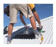
Put a rivet into each corner on the high side of the Soaker Tray, and every 2nd corrugation, fixing the Soaker Tray to the roof sheeting.
