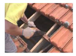
On the roof, you will see where you have pushed back your tile. Remove tiles from this area of the roof and cut out the tile batten. This is only used to support the tiles, that you have now removed.
